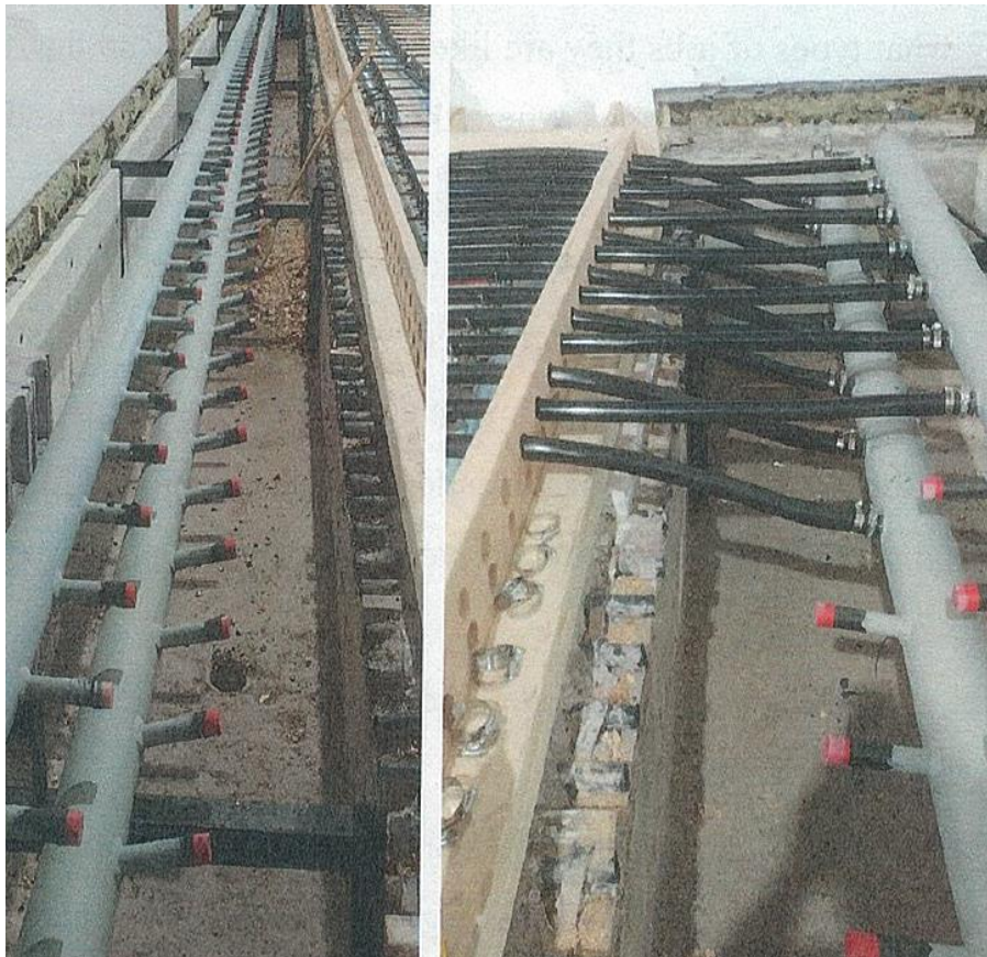
New header pipes in the trench:
